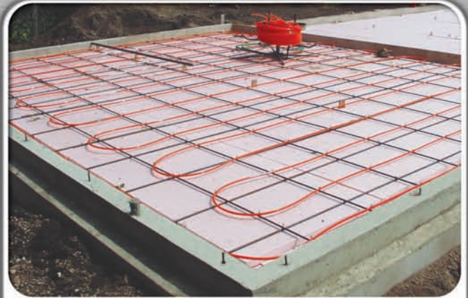
Radiant Heat Single Zone, 8-Loop
